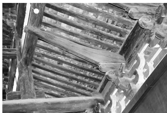
(4) 裳階背面斗拱尾垂木尻
